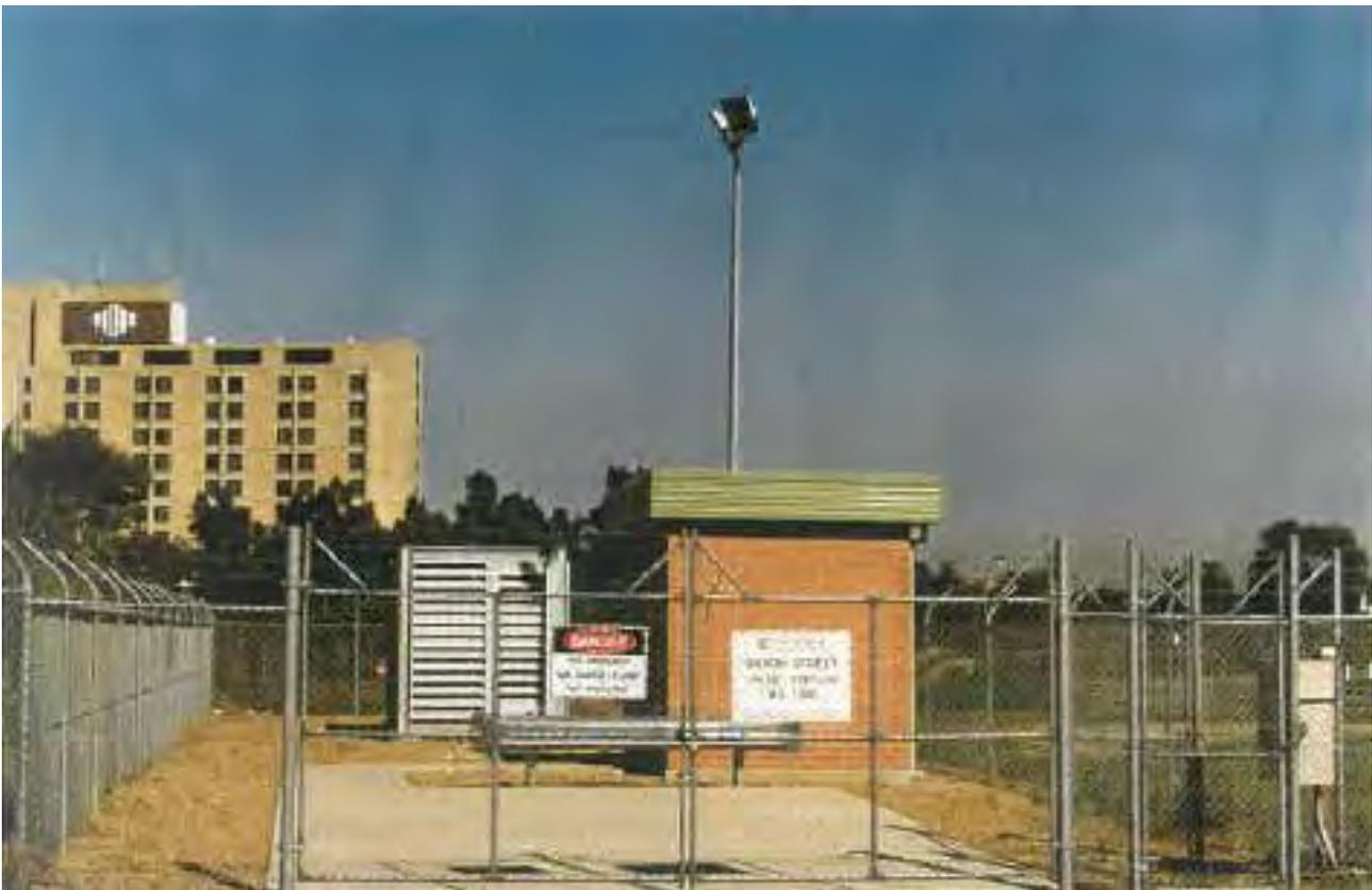
**Figure 6: Above ground valve station and enclosure**
